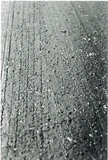
FIG. X1.6 High-Severity Bleeding
