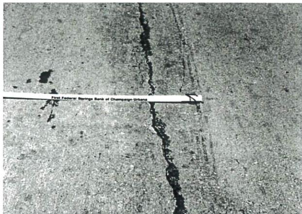
FIG. X2.23 Medium-Severity Linear Cracking
