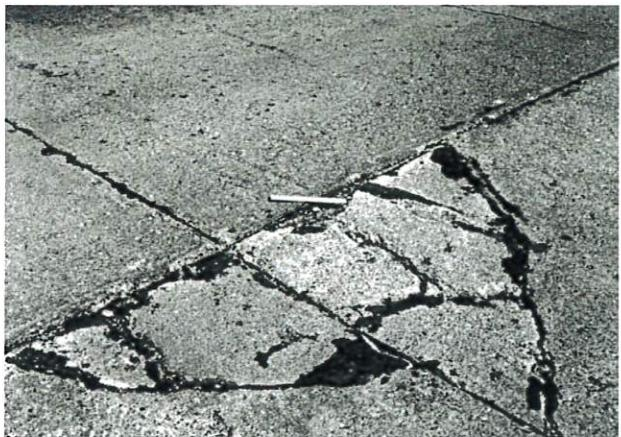
FIG. X2.6 High-Severity Corner Break
