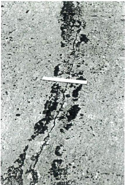
FIG. X2.22 Low-Severity Linear Cracking
