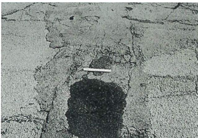
FIG. X1.33 High-Severity Patching and Utility Cut Patching
