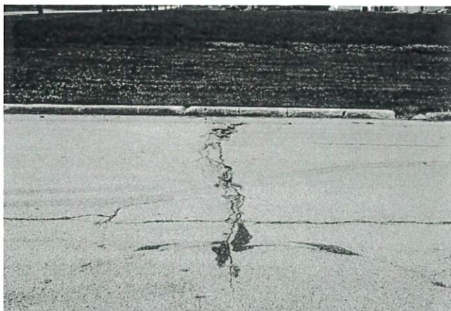
FIG. X1.30 High-Severity Longitudinal and Transverse Cracking
