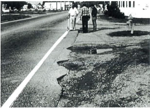
FIG. X1.21 High-Severity Edge Cracking
