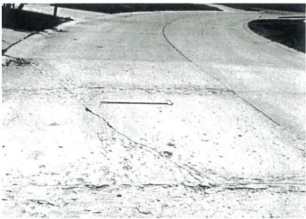
FIG. X2.12 High-Severity Durability Cracking
