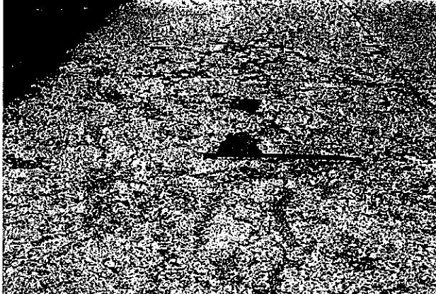
FIG. X2.43 High-Severity Scaling, Map Cracking, and Crazing
