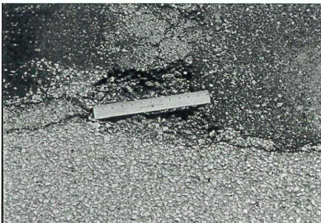
FIG. X1.35 Low-Severity Pothole
