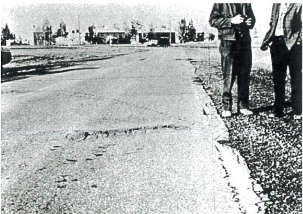
FIG. X1.11 Medium-Severity Bumps and Sags
