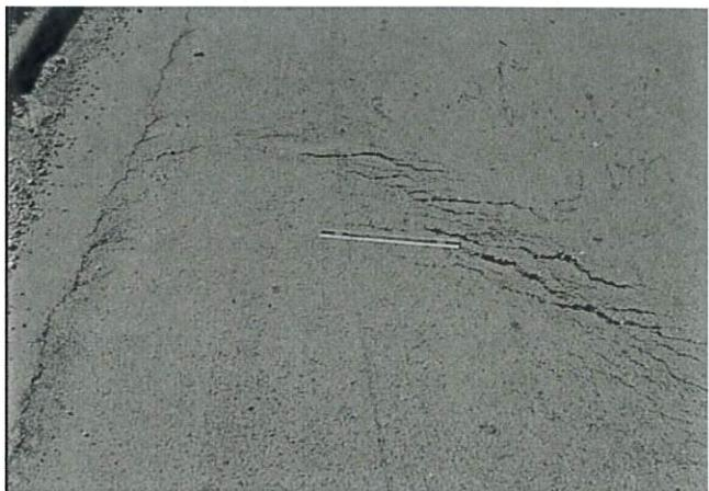
FIG. X1.48 Medium-Severity Slippage Cracking
