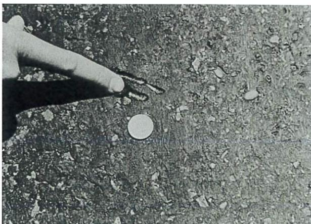
FIG. X1.5 Medium-Severity Bleeding
