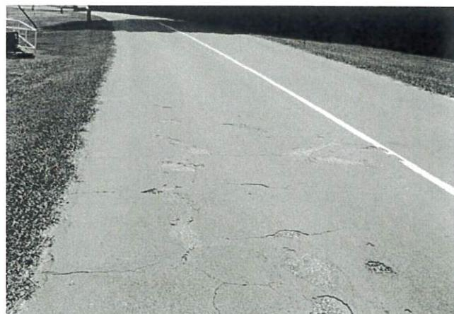
FIG. X1.53 High-Severity Weathering and Raveling
