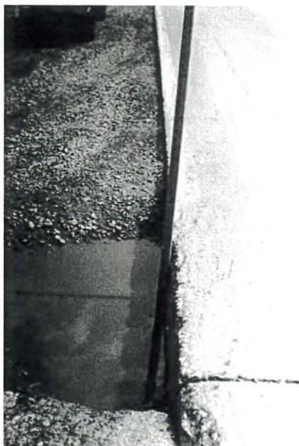
FIG. X2.21 High-Severity Lane/Shoulder Drop-Off
