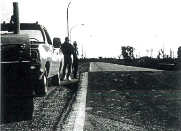
FIG. X2.3 High-Severity Blowup/Buckling
