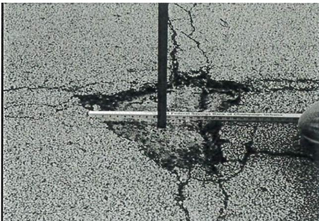
FIG. X1.36 Medium-Severity Pothole
