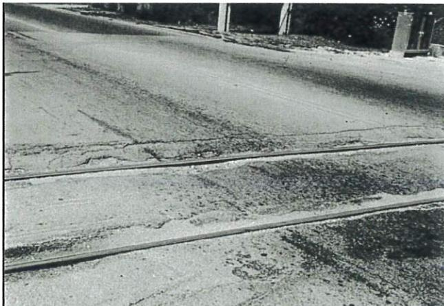
FIG. X1.39 Medium-Severity Railroad Crossing
