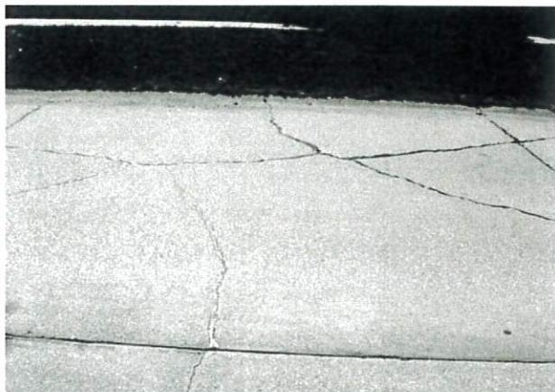
FIG. X2.8 Medium-Severity Divided Slab
