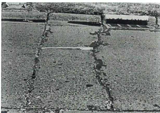
FIG. X2.35 Low-Severity Punchout
