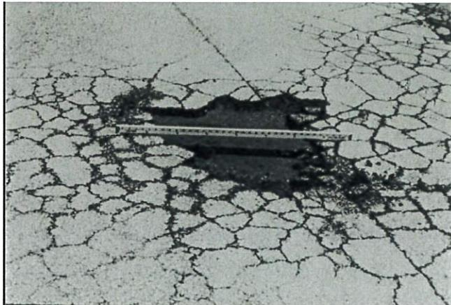
FIG. X1.37 High-Severity Pothole
