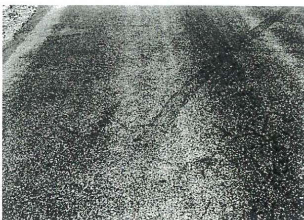
FIG. X1.4 Low-Severity Bleeding
