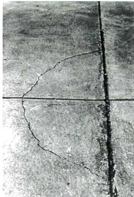
FIG. X2.4 Low-Severity Corner Break
