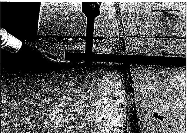
FIG. X2.15 High-Severity Faulting
