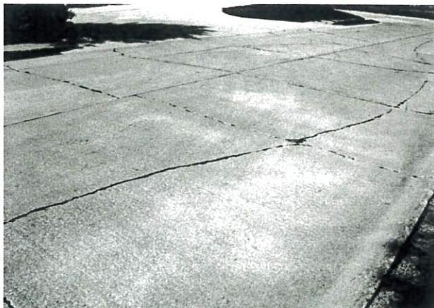
FIG. X2.7 Low-Severity Divided Slab
