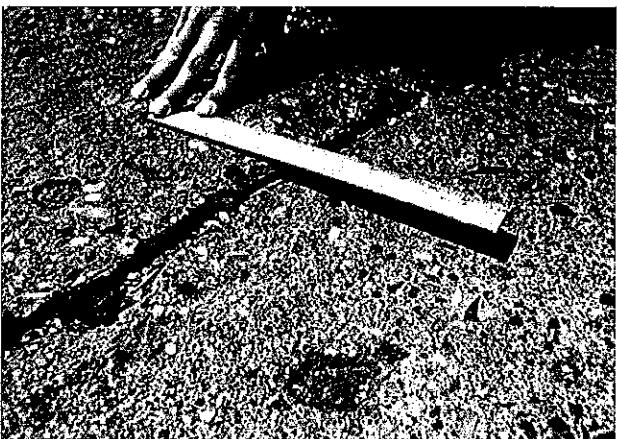
FIG. X2.14 Medium-Severity Faulting
