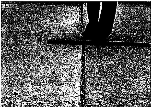
FIG. X2.13 Low-Severity Faulting
