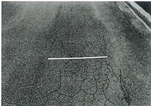
FIG. X1.2 Medium-Severity Alligator Cracking
