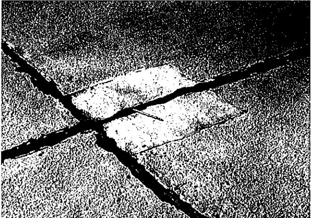
FIG. X2.28 Low-Severity Patching, Small
