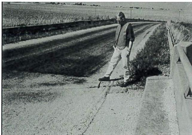
FIG. X1.44 Low-Severity Shoving
