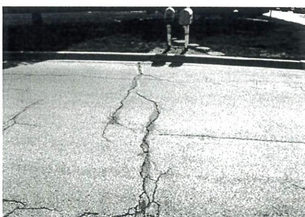
FIG. X1.8 Medium-Severity Block Cracking
