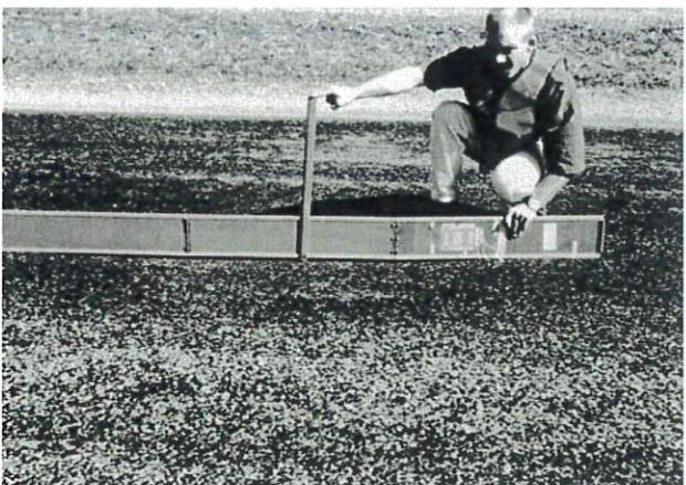
FIG. X1.16 Low-Severity Depression
